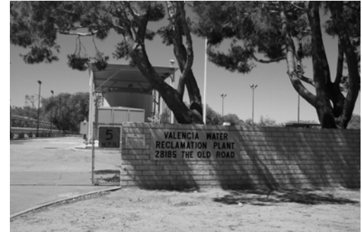
Valencia Water Reclamation Plant
