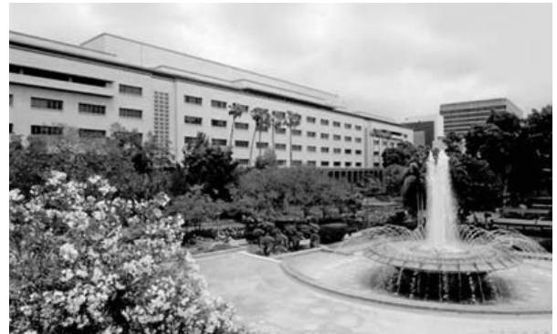
Los Angeles County Hall of Administration
