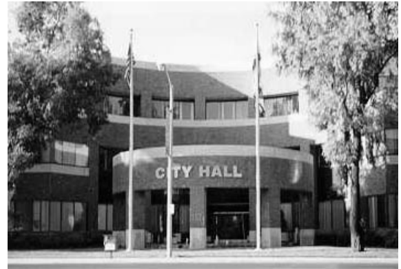
City of Santa Clarita City Hall
