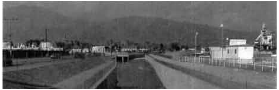
Los Angeles County Flood Control District Facility
